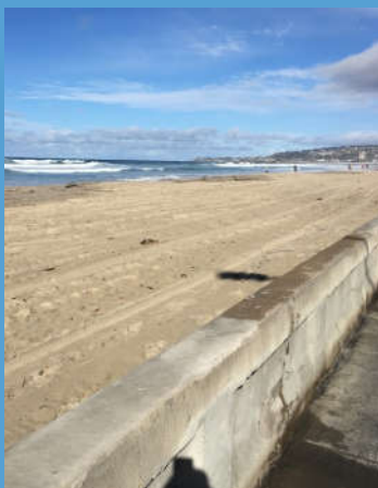
A photo of a seawall in San Diego, CA
