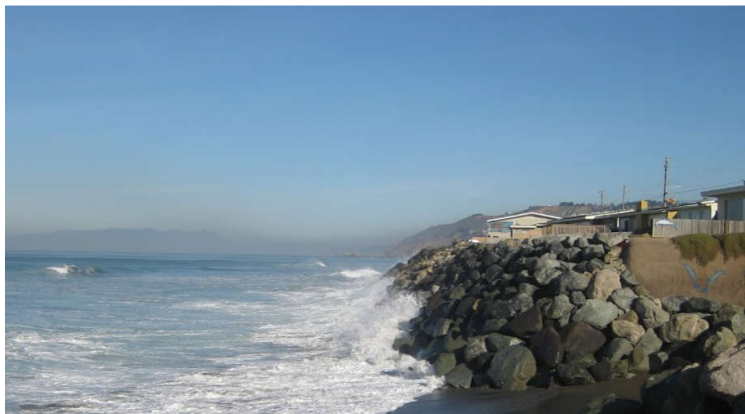
Figure 13: Photo of waves against a revetment in Pacifica, CA
