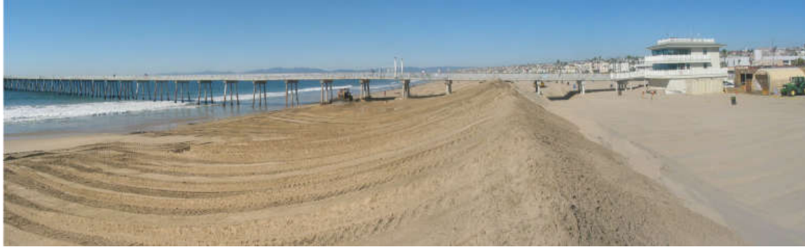
Figure 8: Construction of a temporary winter berm at Hermosa Beach
