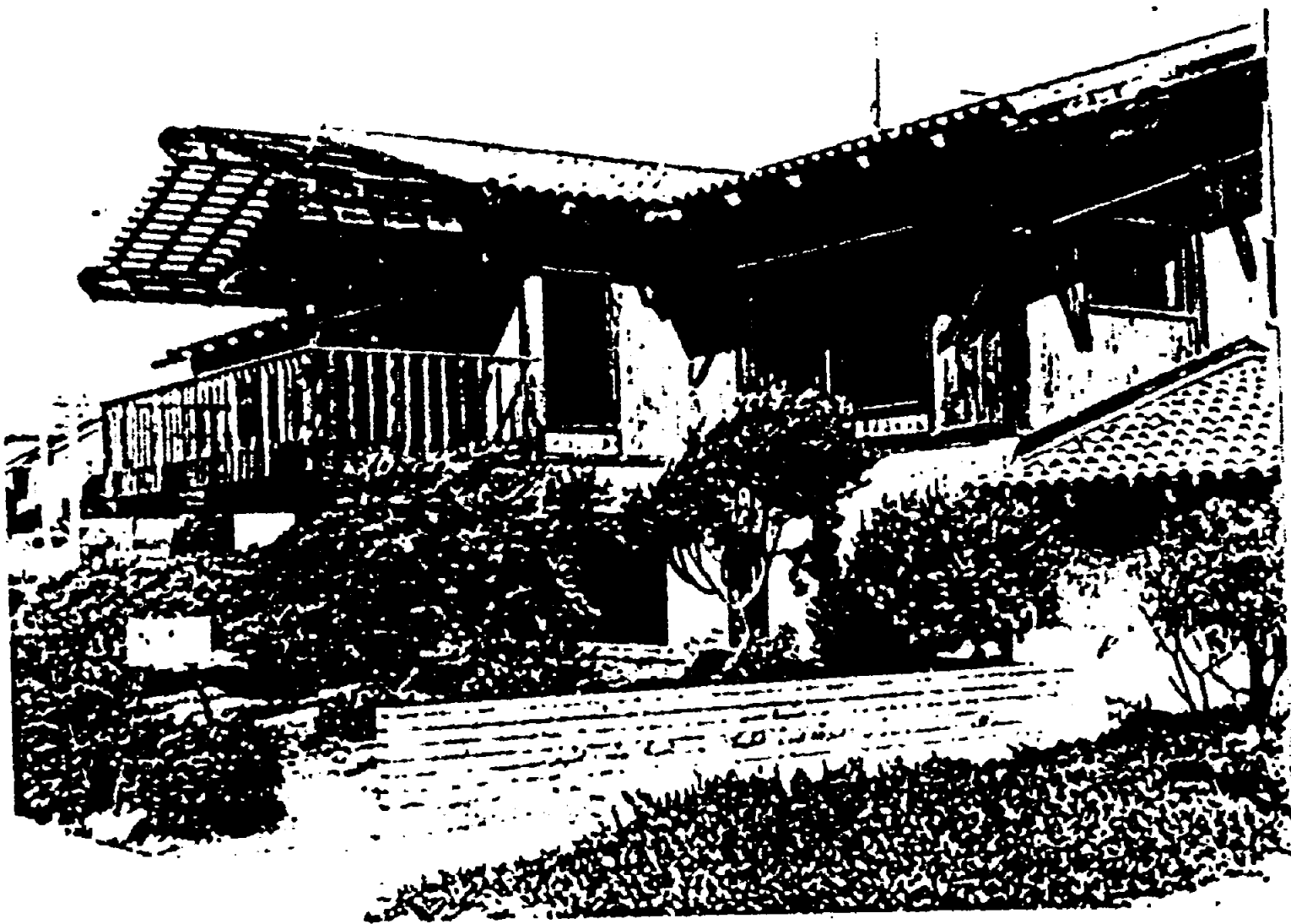
Building at 2600 Strand in Manhattan Beach is now used as office space by County agency; it may have potential for adaptive use for visitor-serving functions.
