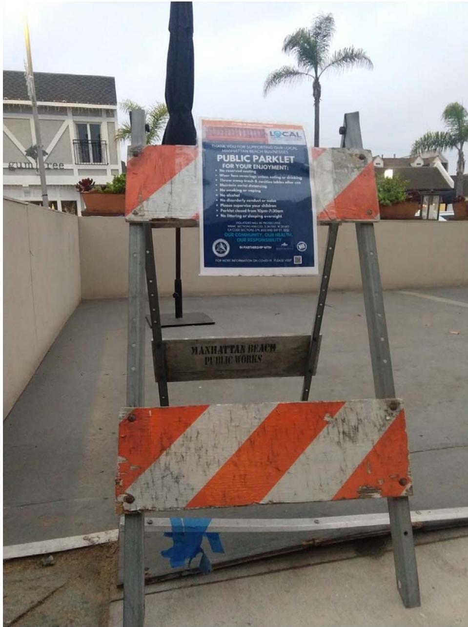
Lower deck trim failure – typical in structures that are reaching end of life
