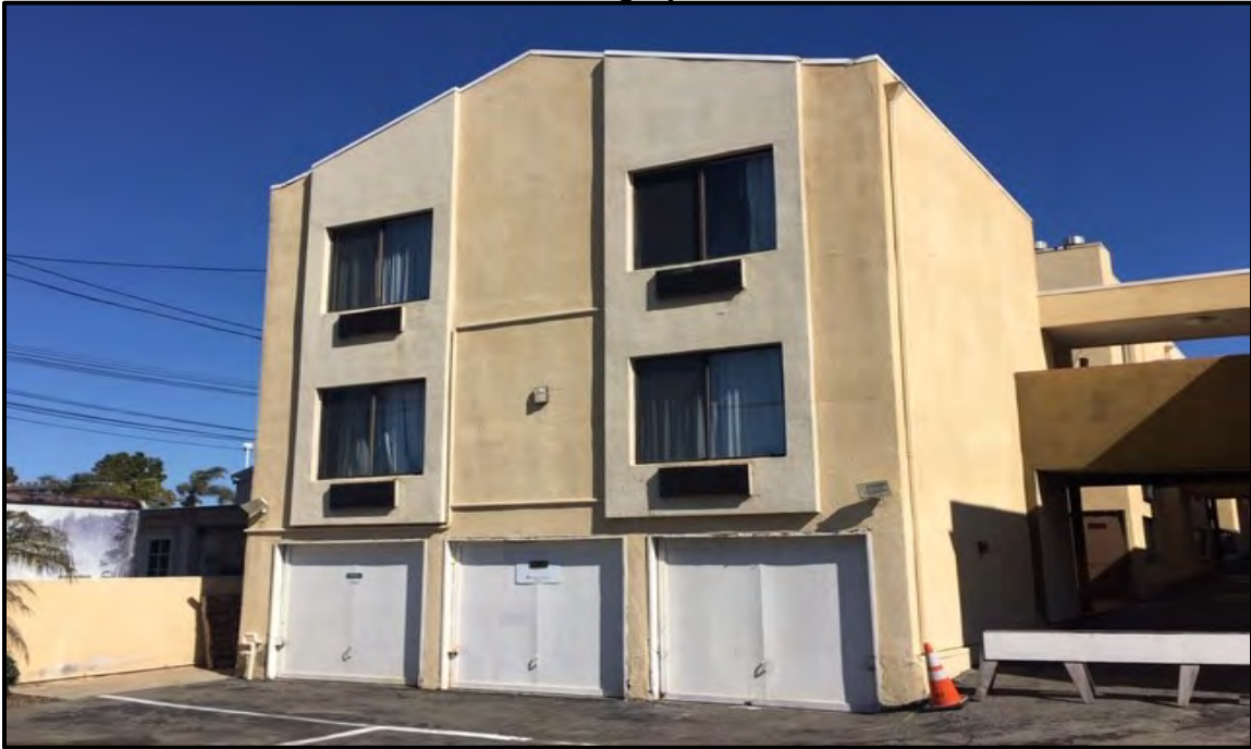
View of hotel (guest rooms and garages) from Melrose Avenue
