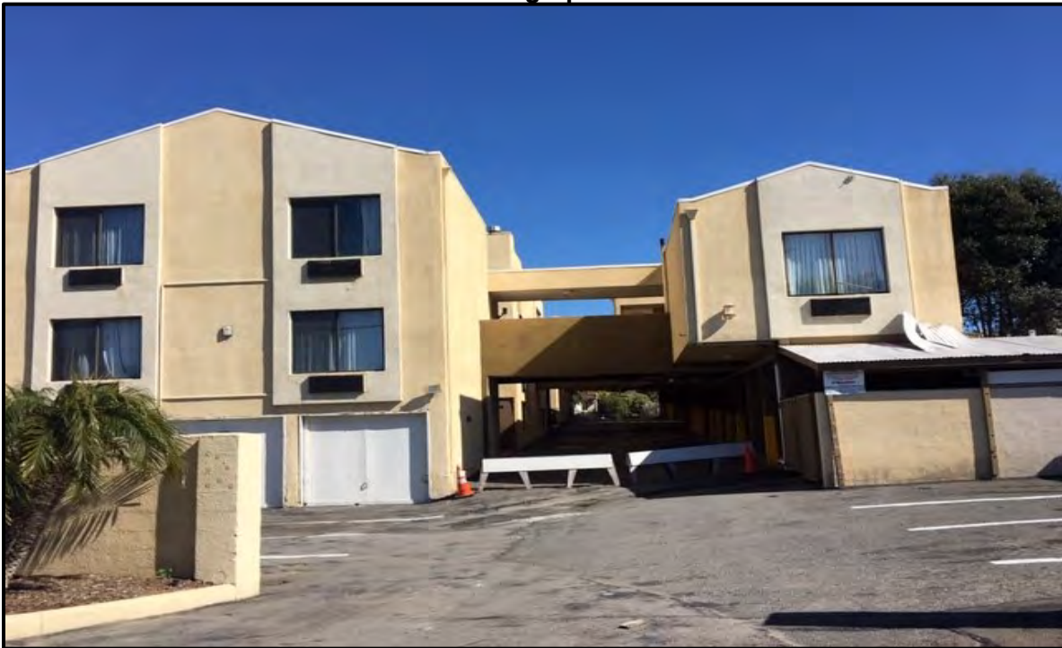
Viewing open parking spaces and access to property from Melrose Avenue
