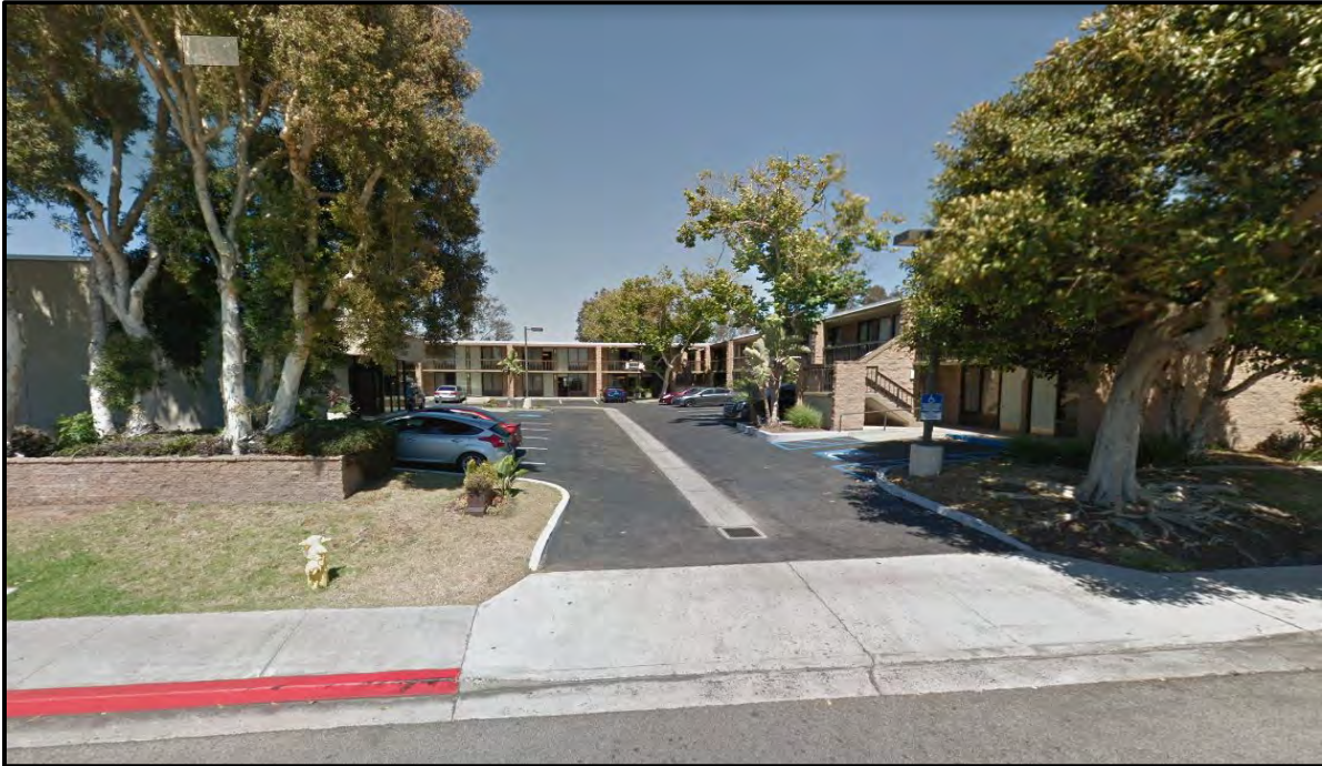
Data 1 Photo – 225 Bay Blvd.
