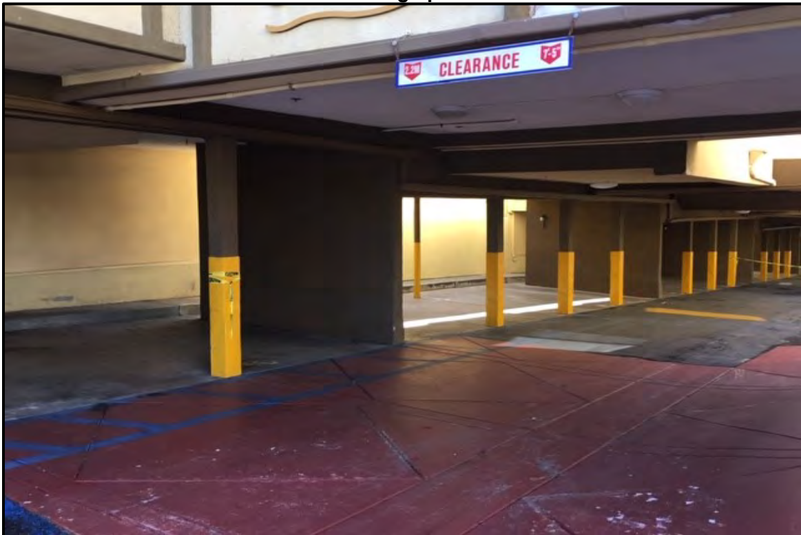
Covered parking stalls under 2 nd floor guest rooms
