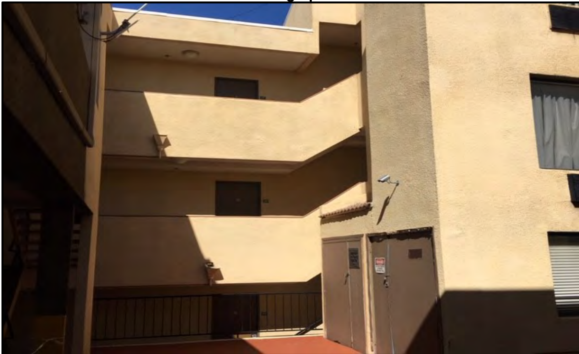
Viewing floor/walkway layout and 3-story design of hotel
