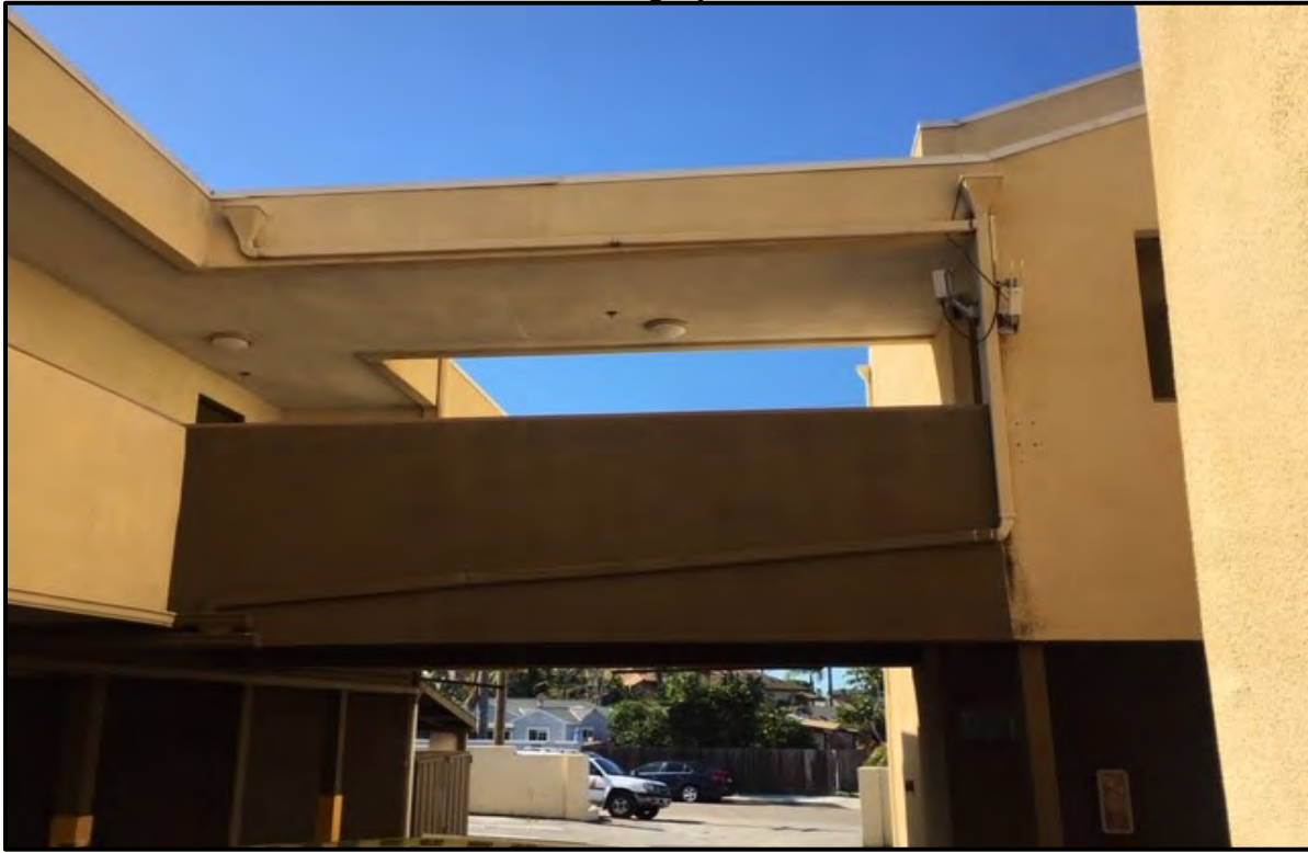
Connecting walkway from north to south side of building Photograph 4
