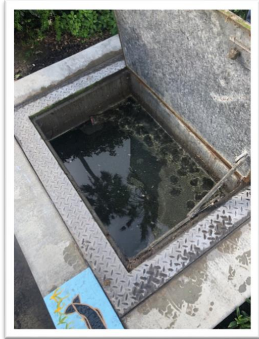
Photo #15 - Inside Strand Stormwater Sump #11 at 43 rd Street
