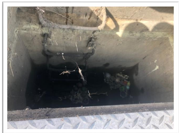
Photo #10 - Inside Strand Stormwater Sump #8 at 28 th Street
