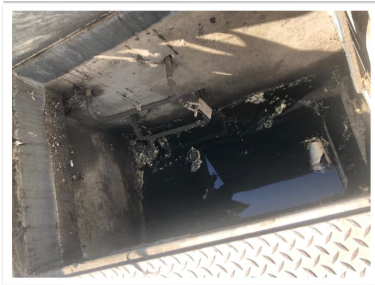
Photo #3 - Inside Strand Stormwater Sump #2 at 6th Street
