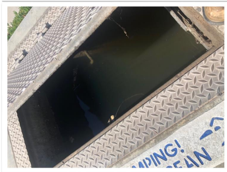
Photo #6 - Inside Strand Stormwater Sump #4 at 8th Place
