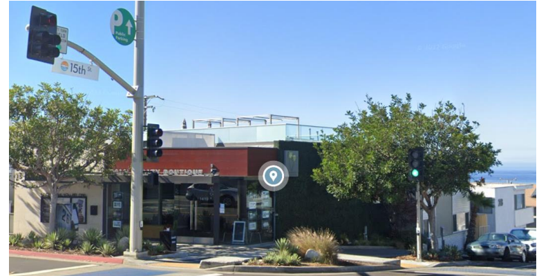
1) Office use at 1419 Highland Ave
