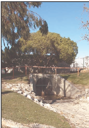
This storm drain outlet feeds water into Polliwog Pond.
