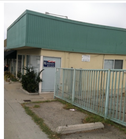
Older single-story commercial building with deferred maintenance and low site utilization.
