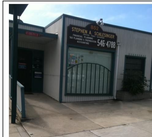
Older commercial buildings showing low site utilization.
