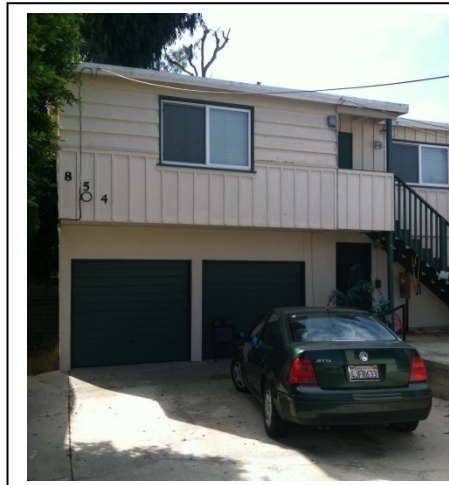
Older, functionally obsolete multi-family building.
