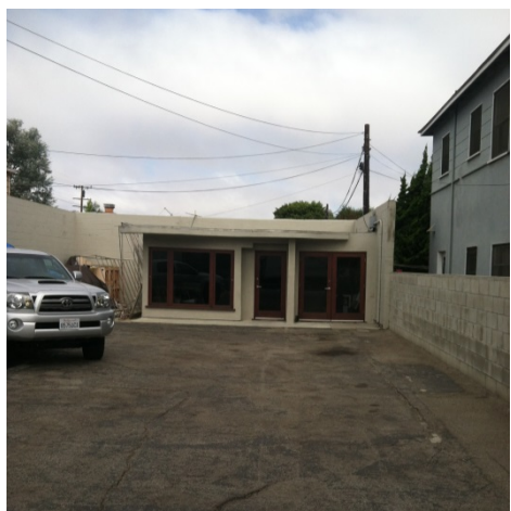
Very low site utilization and disrepair.
