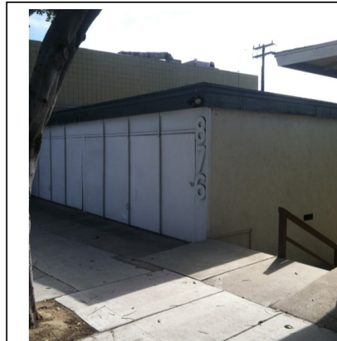
Functionally obsolete building with underutilized capacity.
