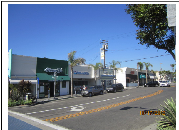
Older single-story commercial buildings on Manhattan Ave. where 3-story residential and mixed-use is permitted.
