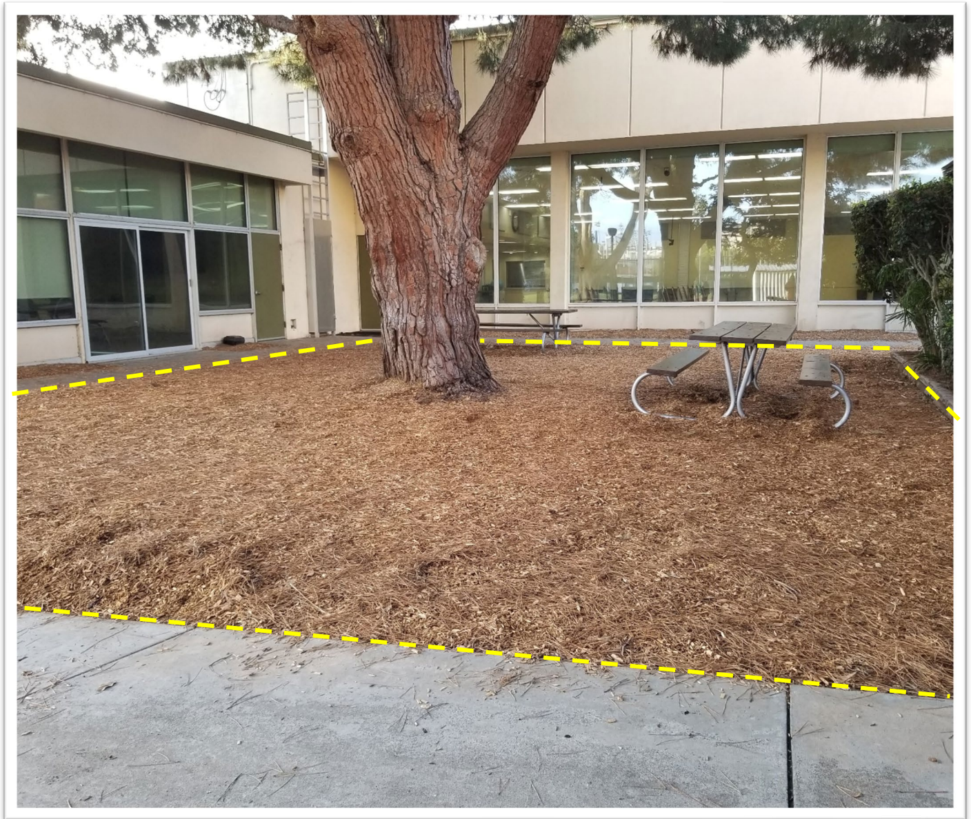
Image 4. Showing the proposed tree protect zone, which should utilize as much of the existing mulch-filled growth space as possible. This area already encompasses the critical root zone. Install protective fencing and restrict the use of construction equipment. Refer to Appendix C for specifications.
