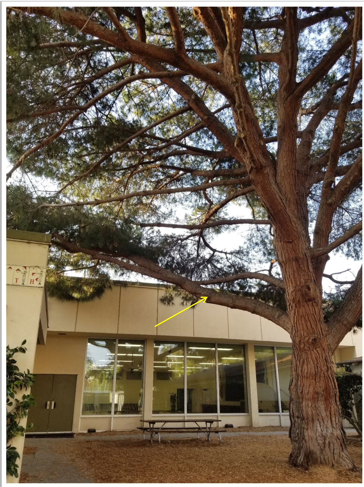
Image 2. Showing the subject tree as seen looking south. Note the limb hanging low over the eastern portion of the community building. Per onsite discussions with city staff, it is recommended that this branch be removed prior to the start of construction activities.
