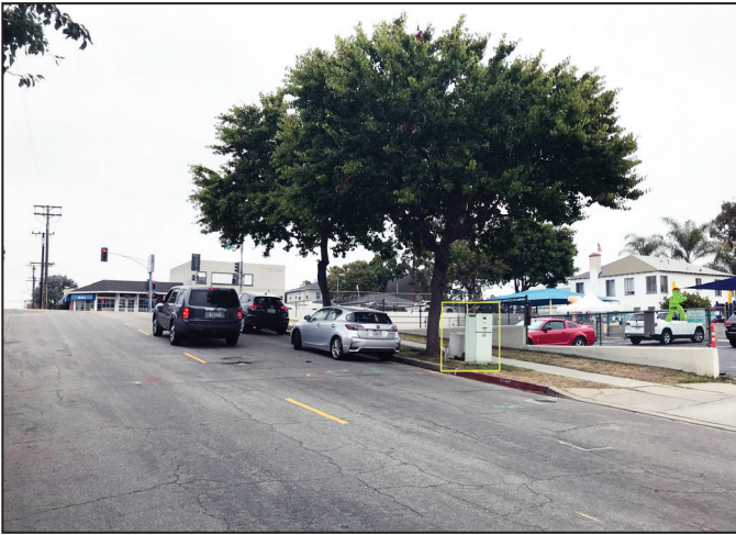
1. View of the Poinsettia Lift Station site.
