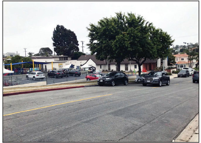
4. View of the east side of Poinsettia Avenue.
