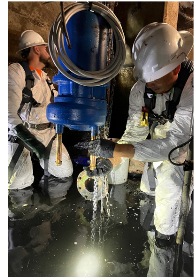
Crew installing new pump at 23rd & Peck pumping station
