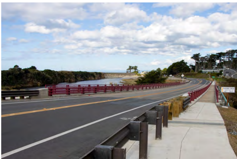
The new Pudding Creek Bridge in Fort Bragg.
