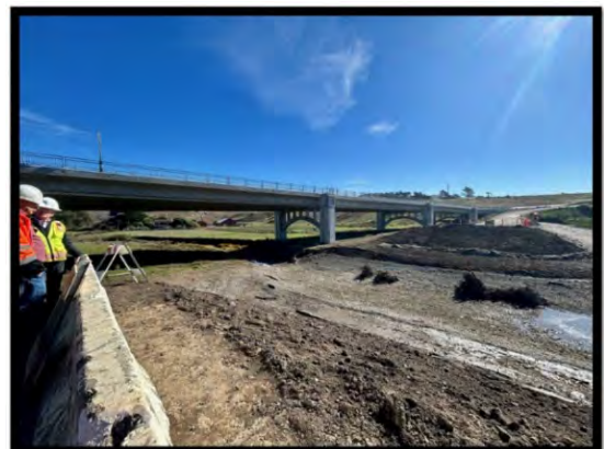
Scotty Creek Bridge.
