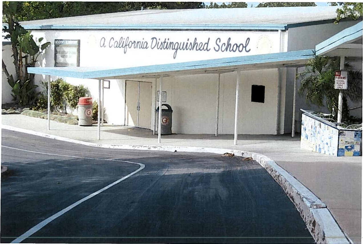
New Loading Zone Turnout
