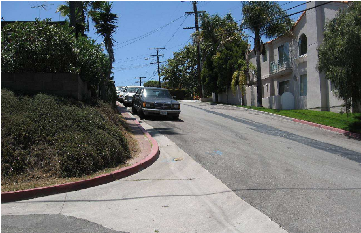
27 th Street at Laurel Avenue Looking Westbound (from South Leg)
