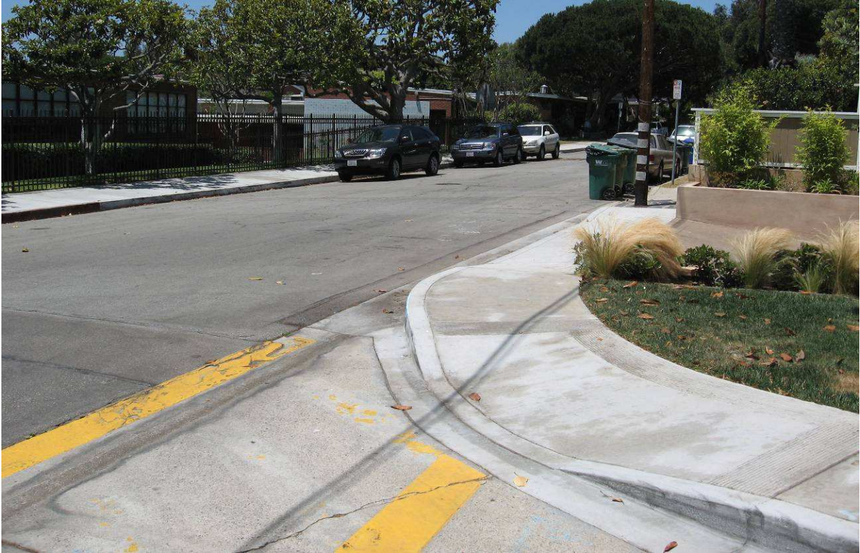
Laurel Avenue at 17 th Street Looking North (From East Leg)
