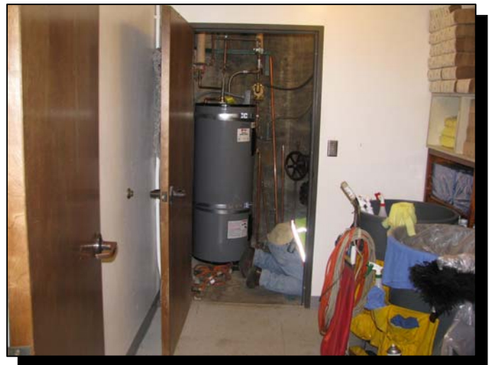
Photograph 6-27 Civic Center Pump Station Access
