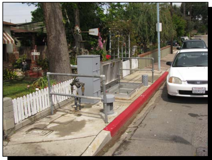
Photograph 6-6 Palm Avenue Pump Station Access
