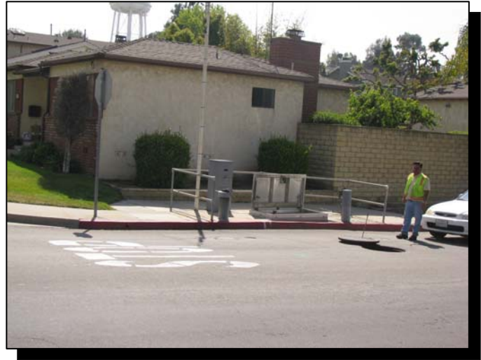
Photograph 6-19 Meadows Avenue Pump Station Access
