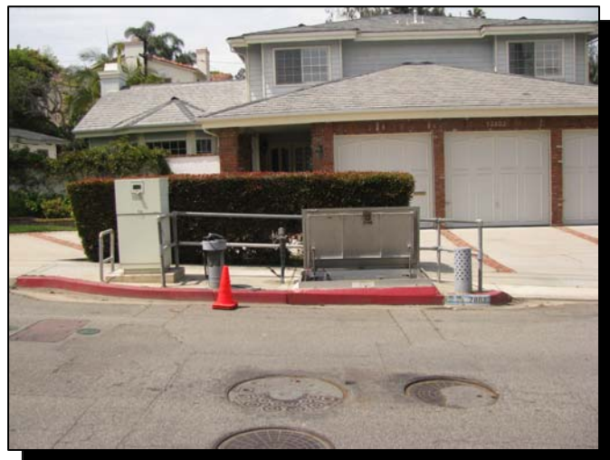
Photograph 6-11 Pacific Avenue Pump Station Access
