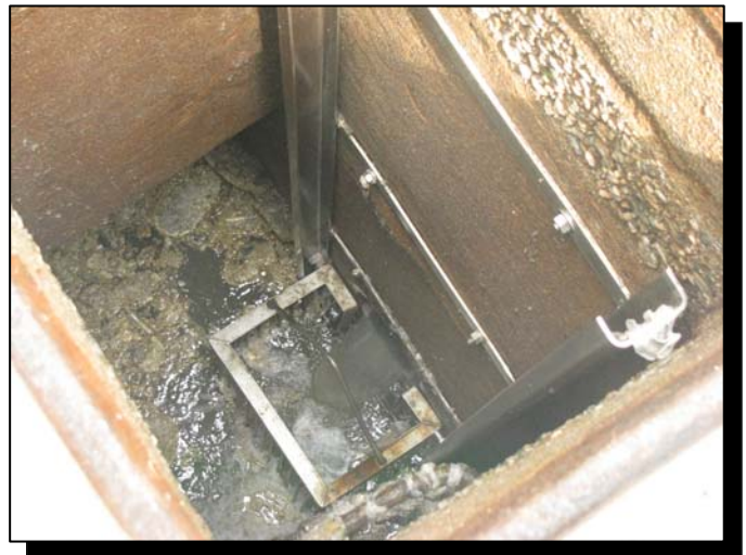
Photograph 6-2 Bell Avenue Pump Station Wet Well
