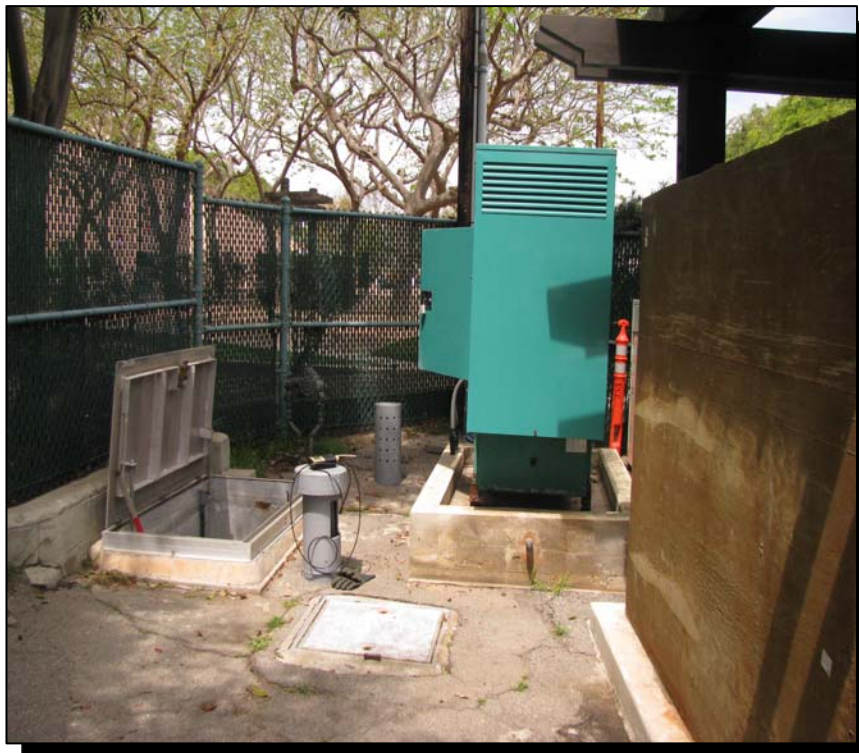
Photograph 6-1 Bell Avenue Pump Station Access
