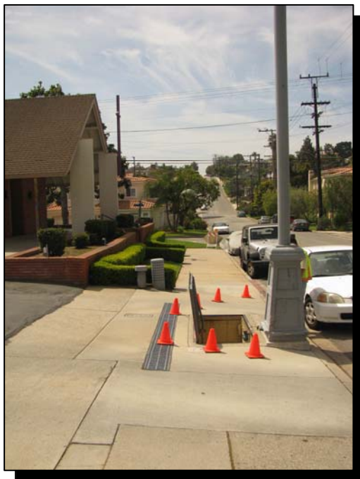
Photograph 6-15 Poinsettia Avenue Pump Station Access
