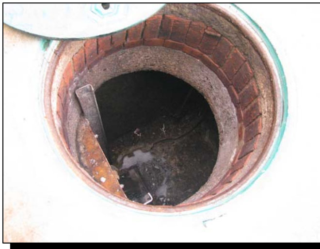
Photograph 6-24 Voorhees Avenue Pump Station Wet Well
