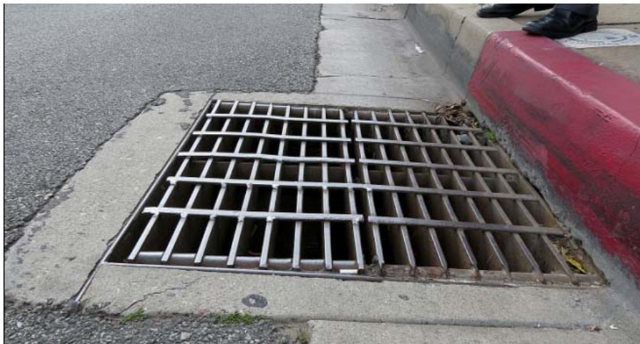
Figure 8 Existing drainage grate on Aviation Boulevard at Warfield Avenue
