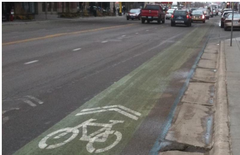
Figure 37 "Super-sharrow" green lane treatment
